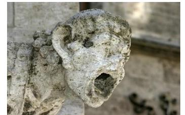
Abb. 2: A gargoyle that has been damaged by acid rain [1]
